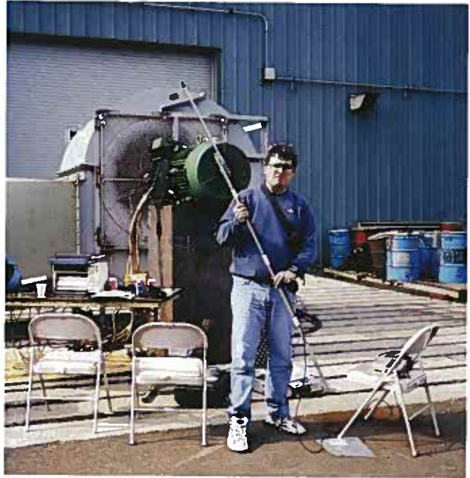
Gambino conducting a performance verification of a subway exhaust fan using high-velocity acoustic measurement tools.
